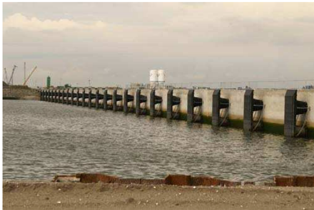
Figure 5: Partly completed quay wall at Rotterdam Europort
