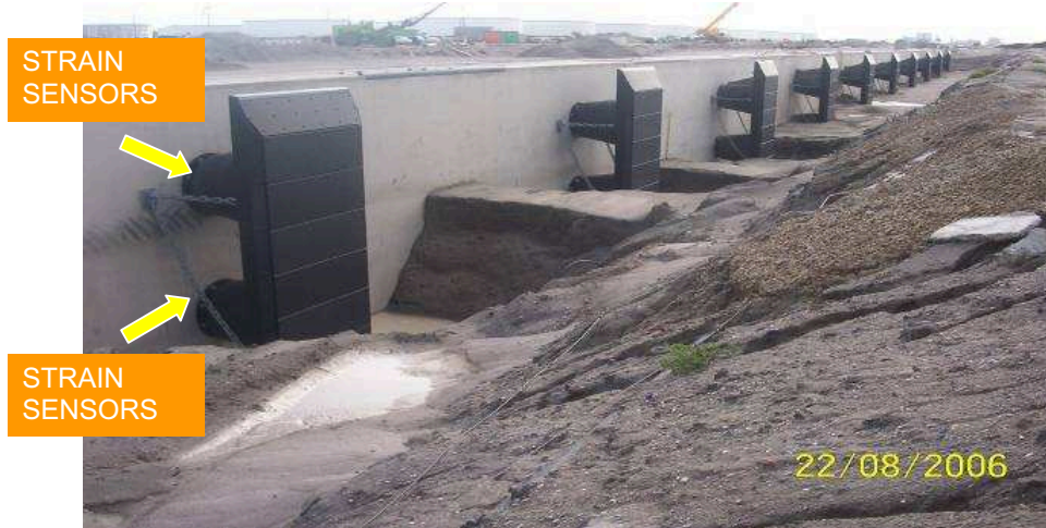
Figure 6: Strain sensors mounted on a series of 24 fenders
