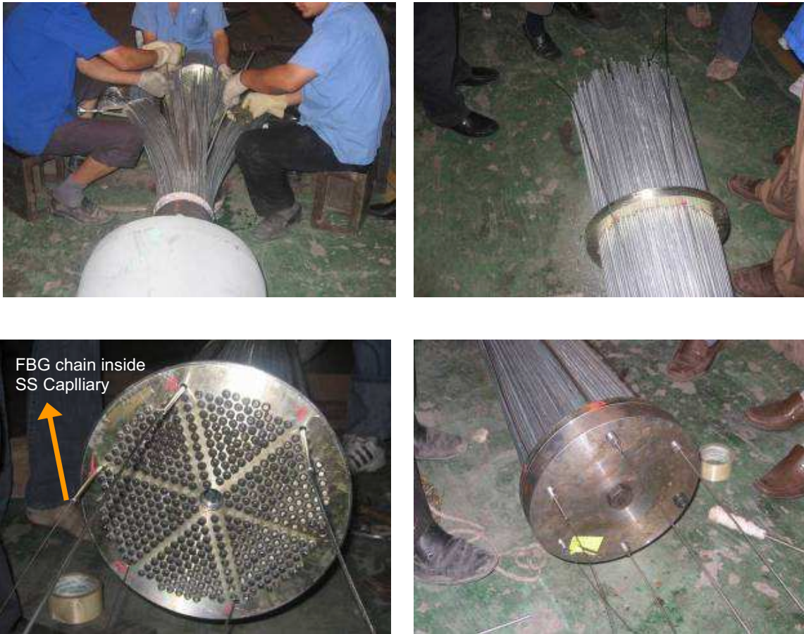
Figure 4: FBG Sensors inside the Stay Cable
