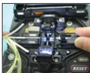
2. Slide splice sleeve over splice point.
